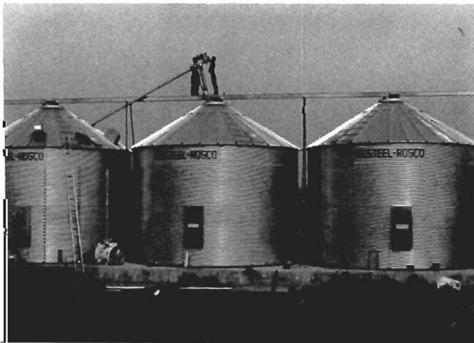
Figure 17. Conveyors and/or Catwalks Supported by the Roof
