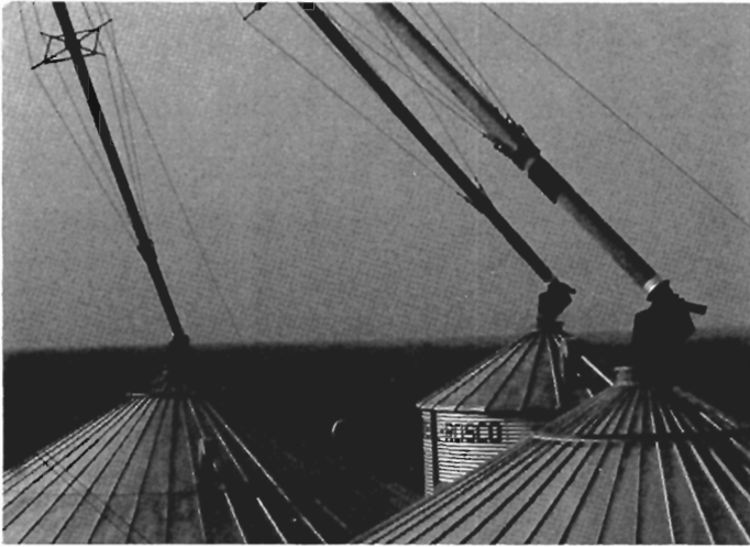
Figure 16. Down Spouts Supported by Roof Cap
