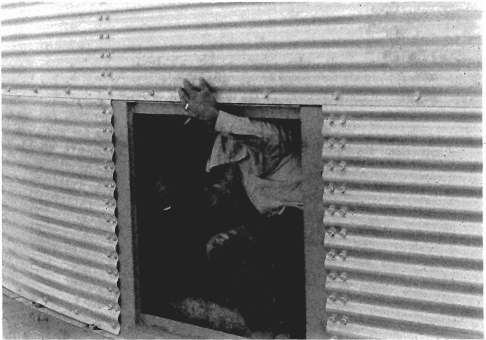
Figure 5. Door Should be Accessible
